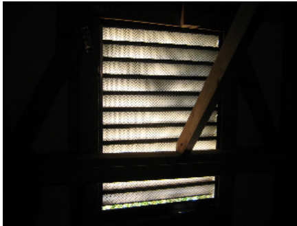
Attic Vent from inside
