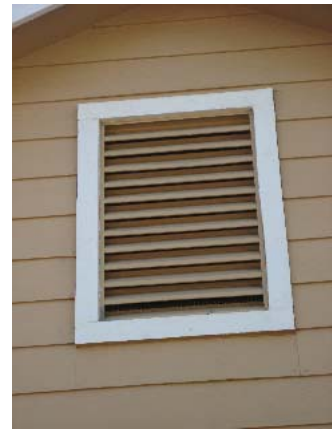
View of Attic Vent from outside
